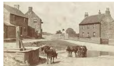
Pump and pond
