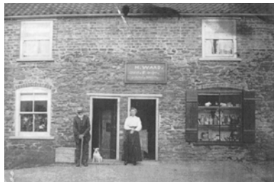
H Ward General Shop
